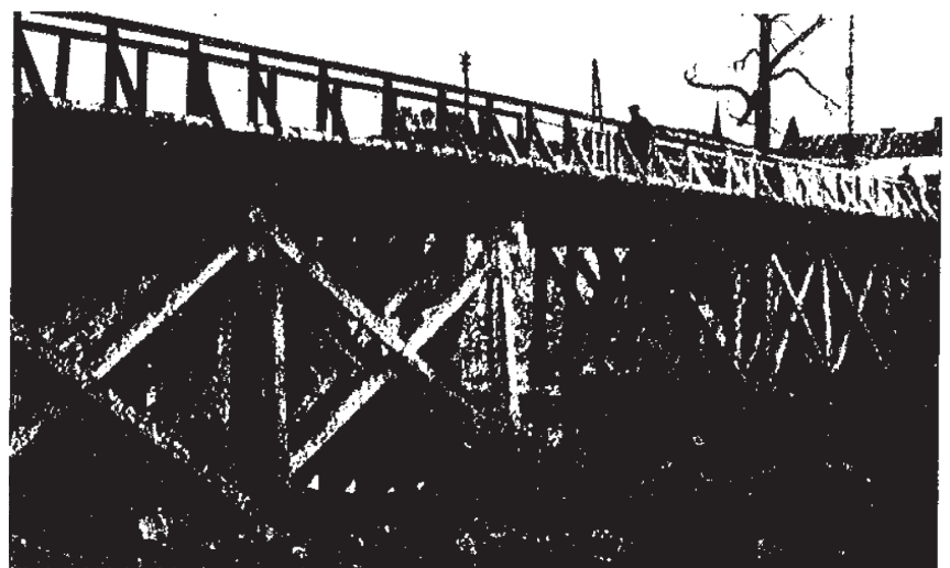
„A“ Company's bridge at Dommeldange Rule, Luxemburg
